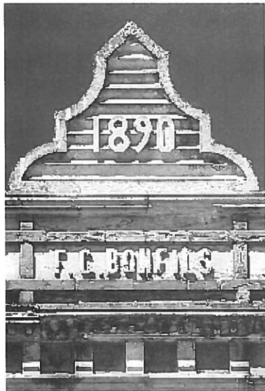
Historic Building Sign at Parapet
