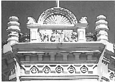
Historic Building Sign at Parapet
