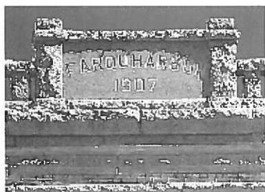
Historic Building Sign at Parapet
